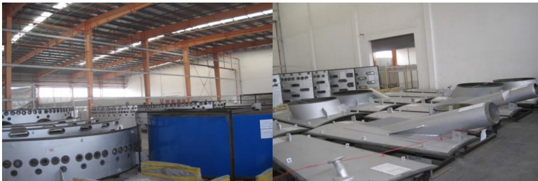
Blast furnace shell
