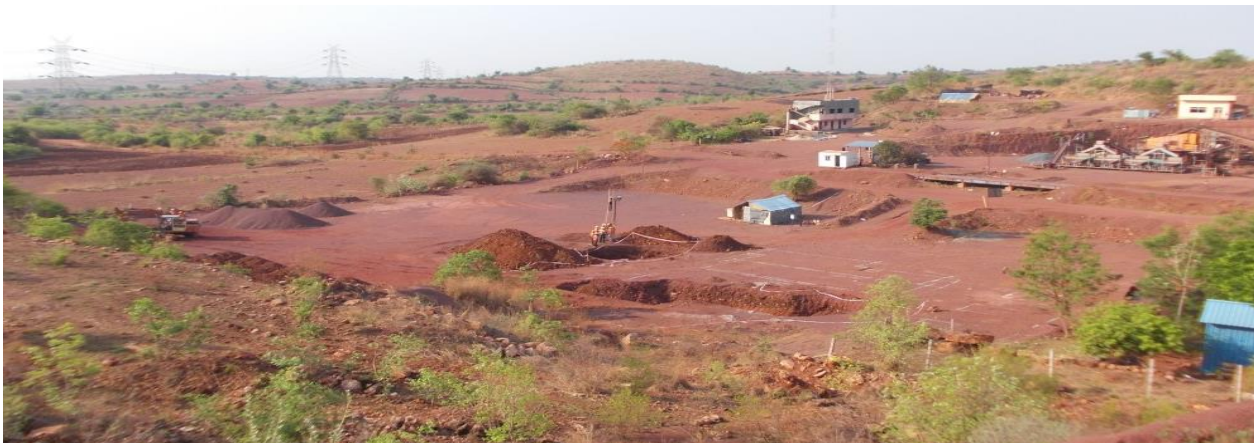
Sequential Site Images Showing Construction Progress
