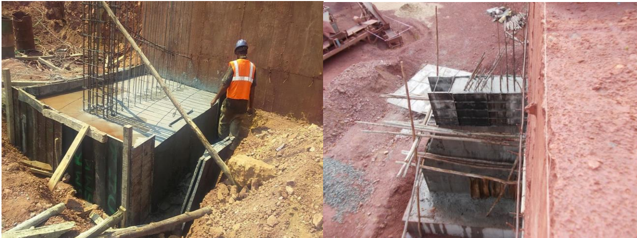
Retaining wall buttress construction
