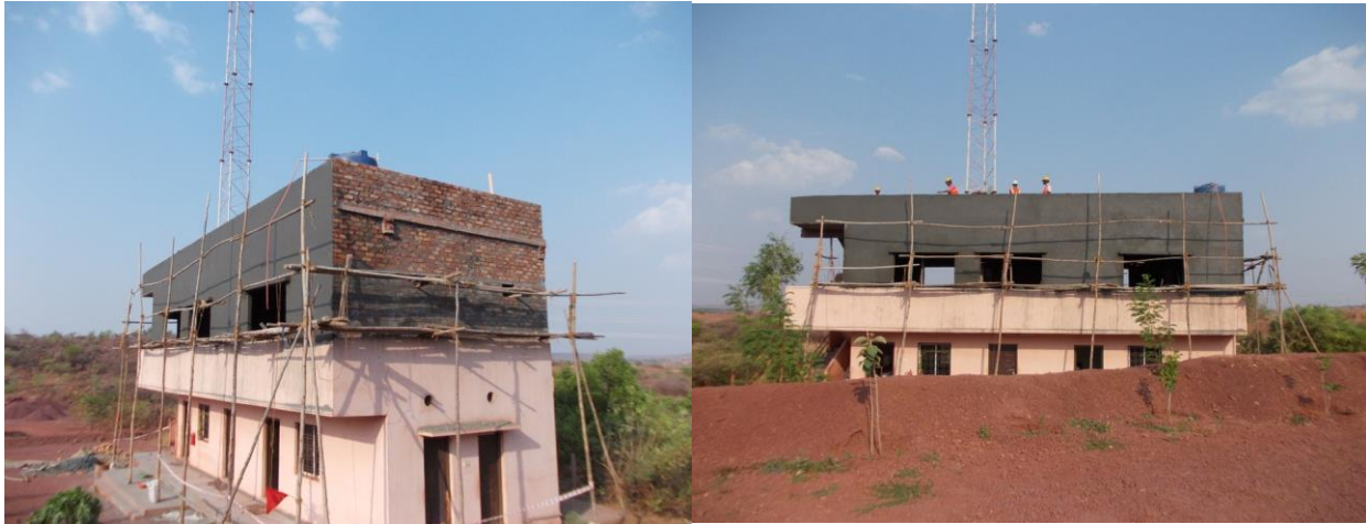
Office second story construction
