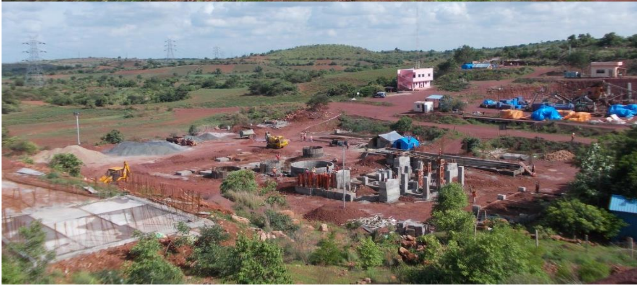
Sequential Site Images Showing Construction Progress
