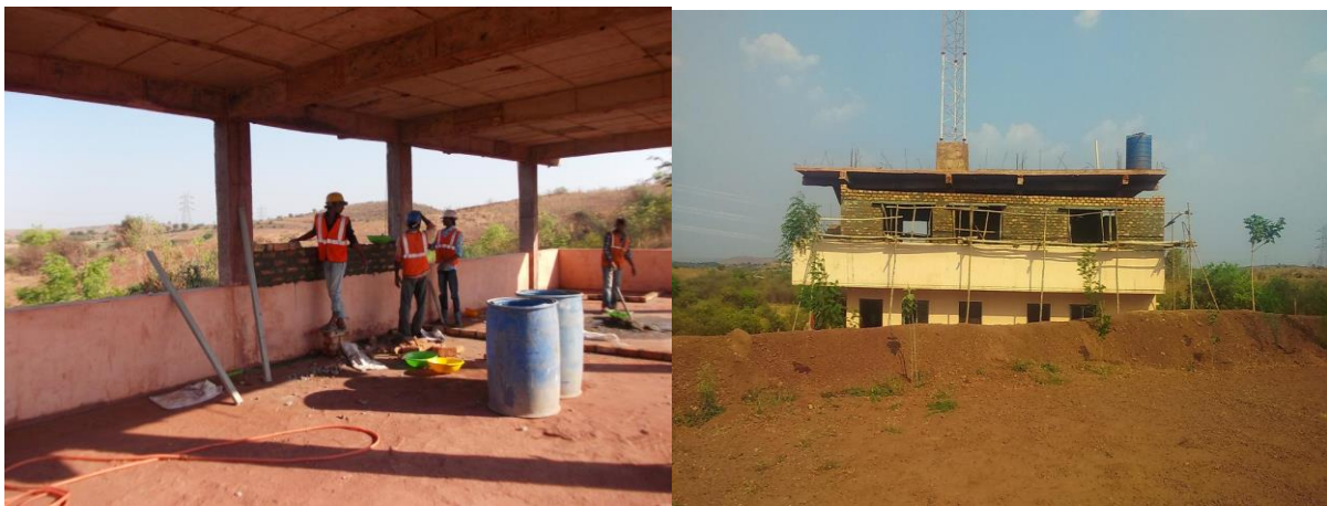
Office second story construction
