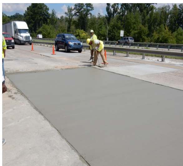
Figure 2 2 nd Field Trial of EdenCrete™ On I-20
