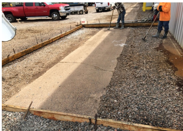
Figure 8. Minimal sub-base preparation for second slab
