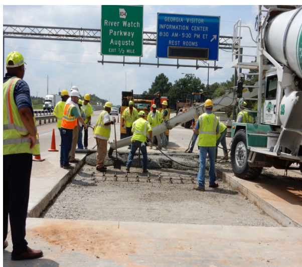
Figure 1 2 nd Field Trial of EdenCrete™ On I-20
