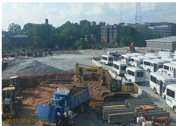
Figure 10. Brady Mobility Facility
