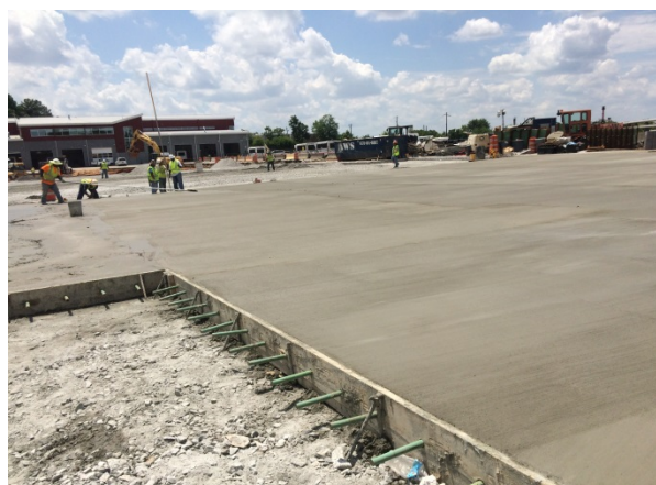
Figure 11. EdenCrete™ enriched slab being installed
