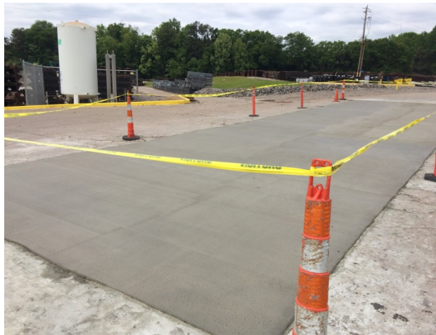
Figure 7. Completed first slab
