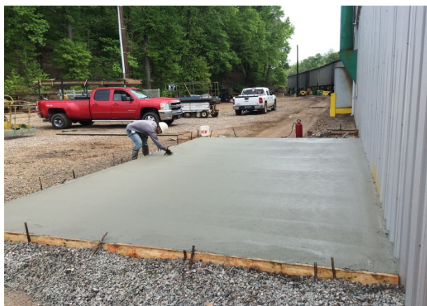
Figure 9. Completed second slab
