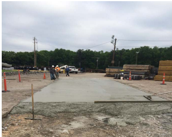
Figure 6. Partially poured first slab
