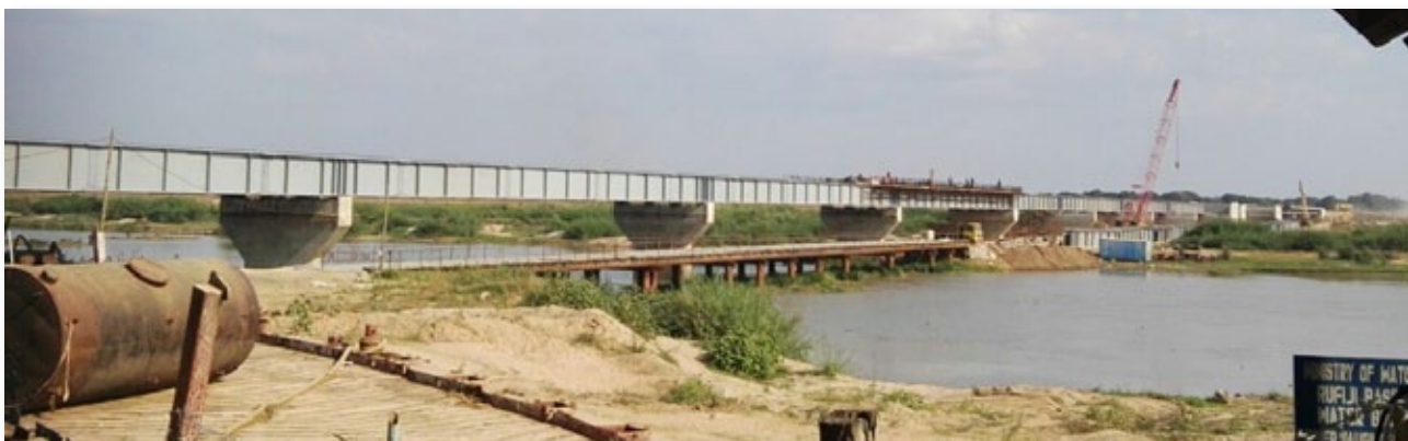
Construction of Kilombero Bridge
