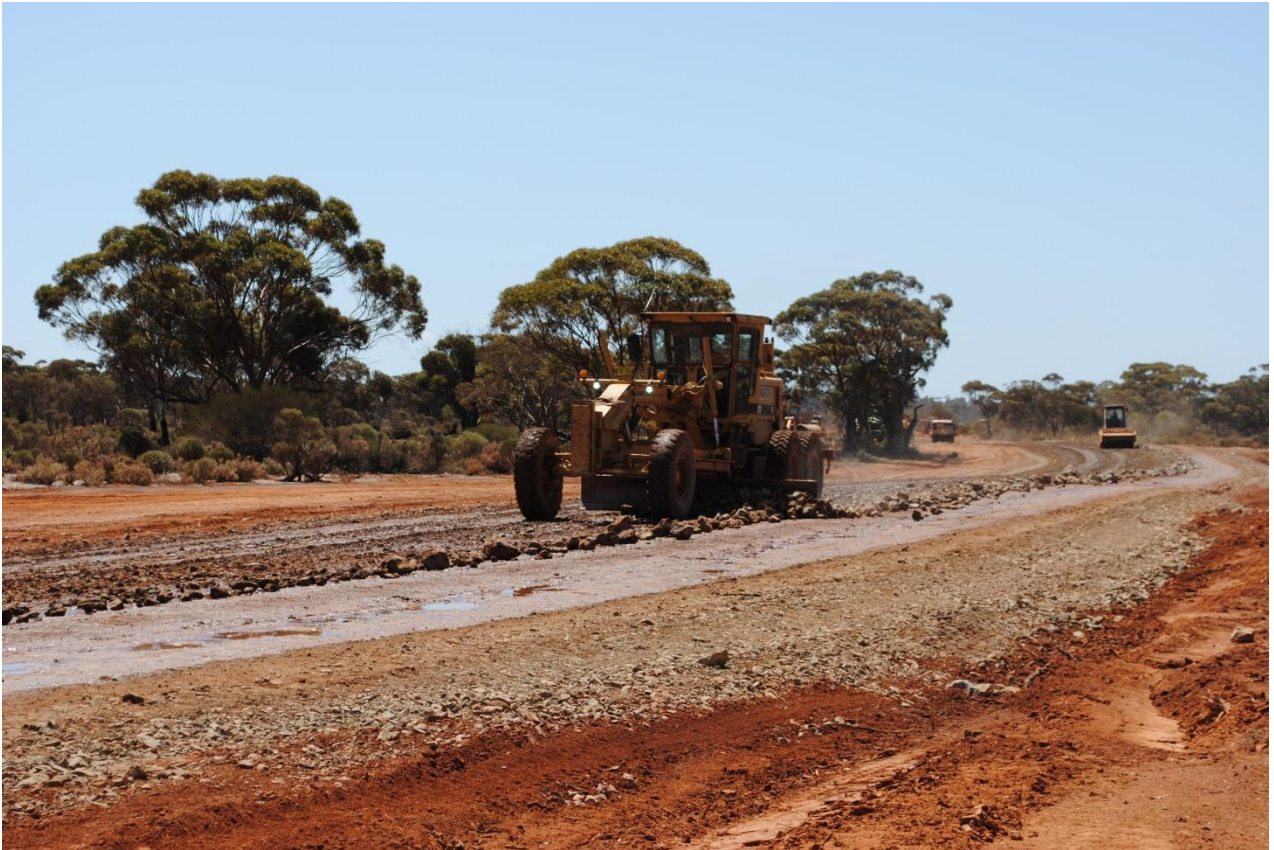
Penny's Find : Road re-alignment under construction
