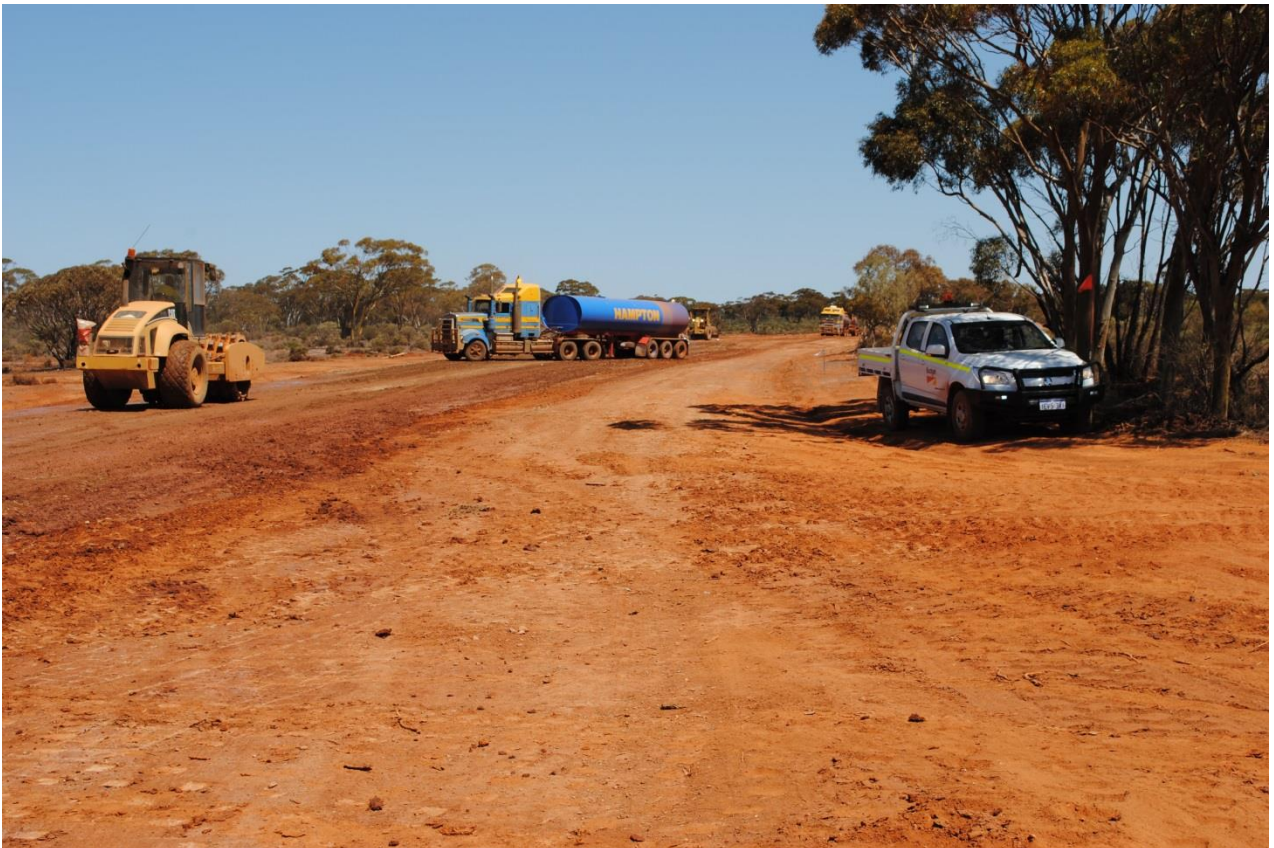
Penny's Find : Road re-alignment under construction
