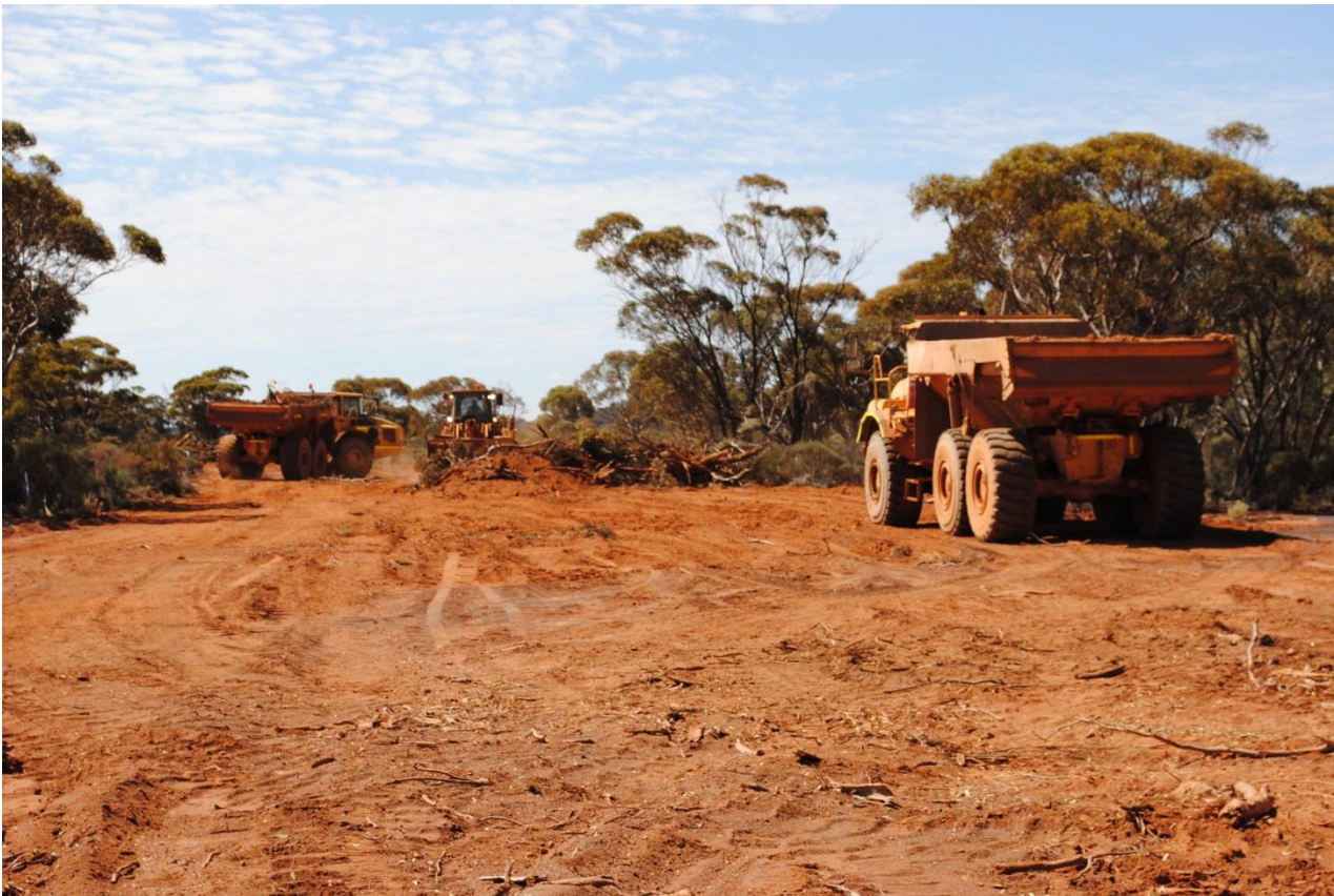
Penny's Find : Road re-alignment clearing
