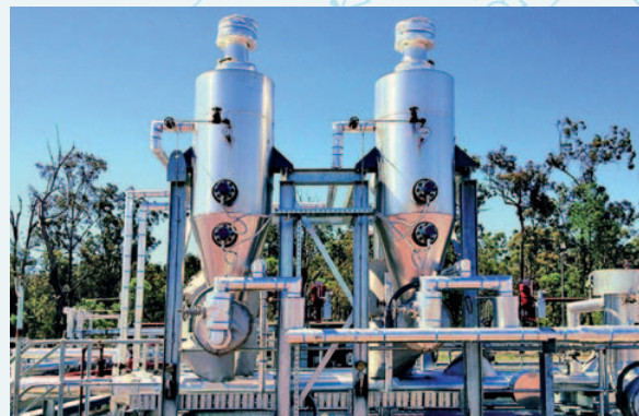
Typical Knock-out Pots used in ISG Demonstration Facilities (Source: Carbon Energy 2012 Annual Report).
