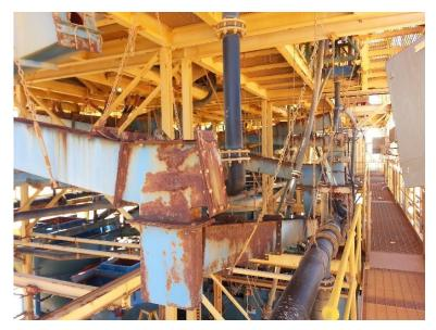
Figure 17 – PCP Launders in Very Poor Condition
