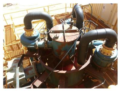
Figure 18 – PCP Tailings Cyclones Showing Significant Corrosion around the Distributor and Launder
