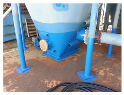
Figure 16 - PCP Sumps Following Site Based Repair
