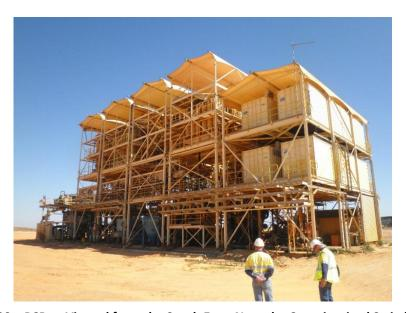
Figure 20 – PCP as Viewed from the South East, Note the Containerised Switchrooms
