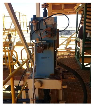
Figure 15 – PCP Samplers Are All in Poor Condition and Have Significant Corrosion
