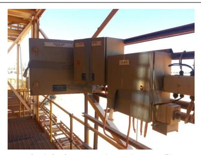
Figure 19 – PCP Electrical and Instrumentation Junction Boxes All in Poor Condition
