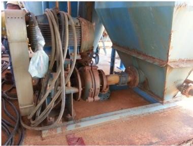
Figure 11 – PCP Pumps All in Reasonable Condition. Electrical Cables Coiled.
