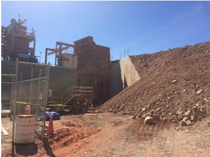
Photo 4: ROM wall constructed and backfilled
