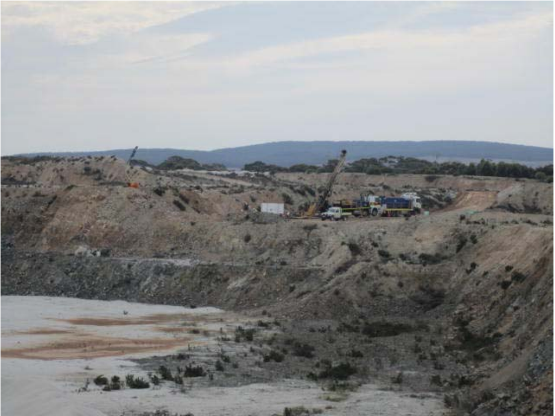
Figure 4: Diamond drilling underway on MTCDD2, Dowling Pit, April 2016
