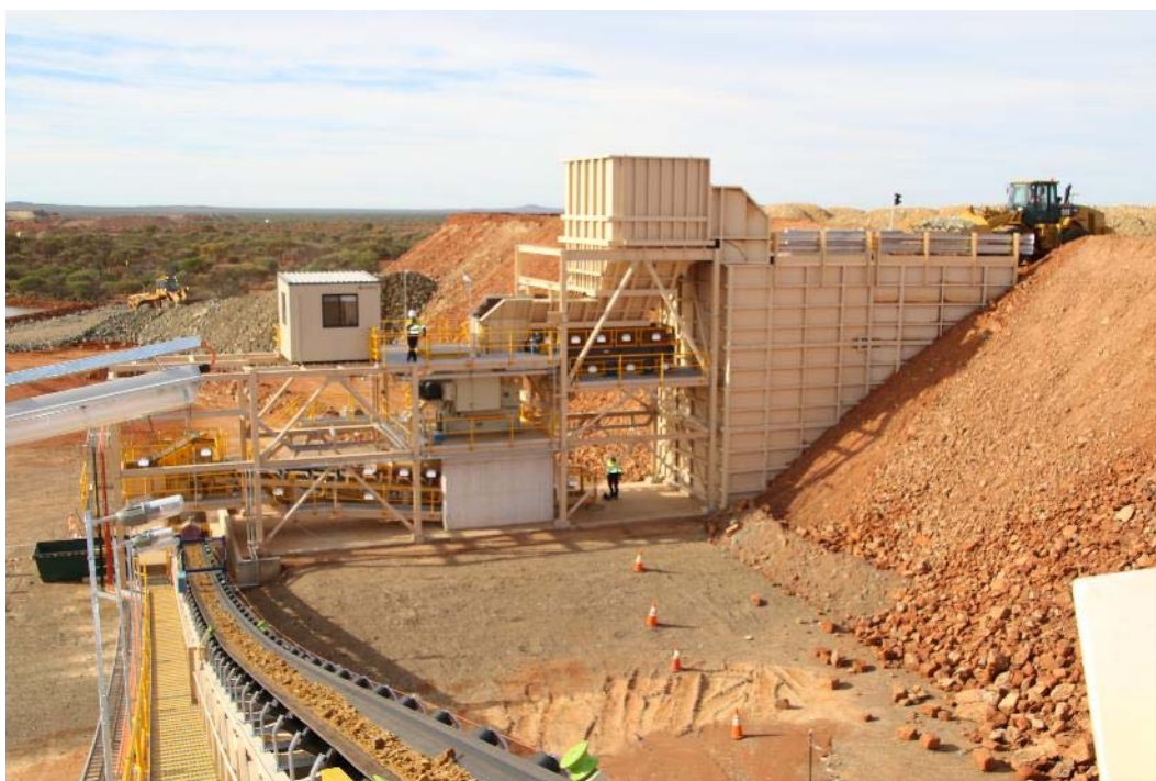
Figure 1. Completed crushing circuit and ROM pad with crushed waste material on conveyor.
