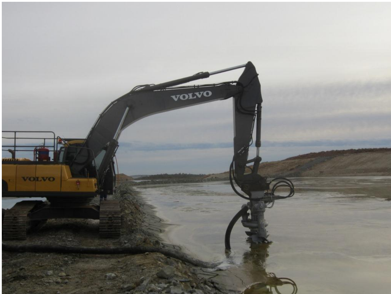
Photograph 3. Gold tails return pump commencing operation
