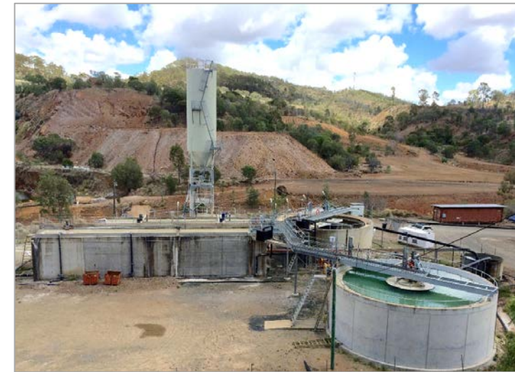
Mount Morgan water Treatment Plant
