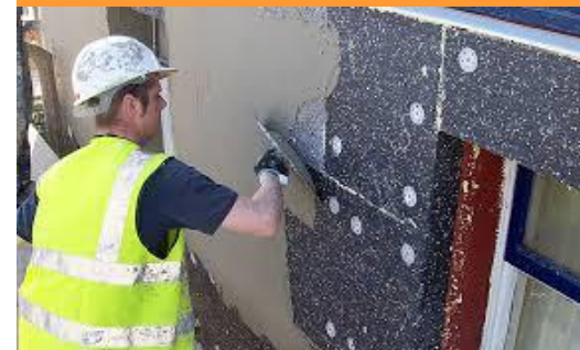
Installing insulation foam
