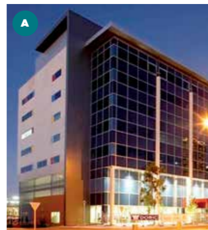
836 WELLINGTON STREET, PERTH WA
