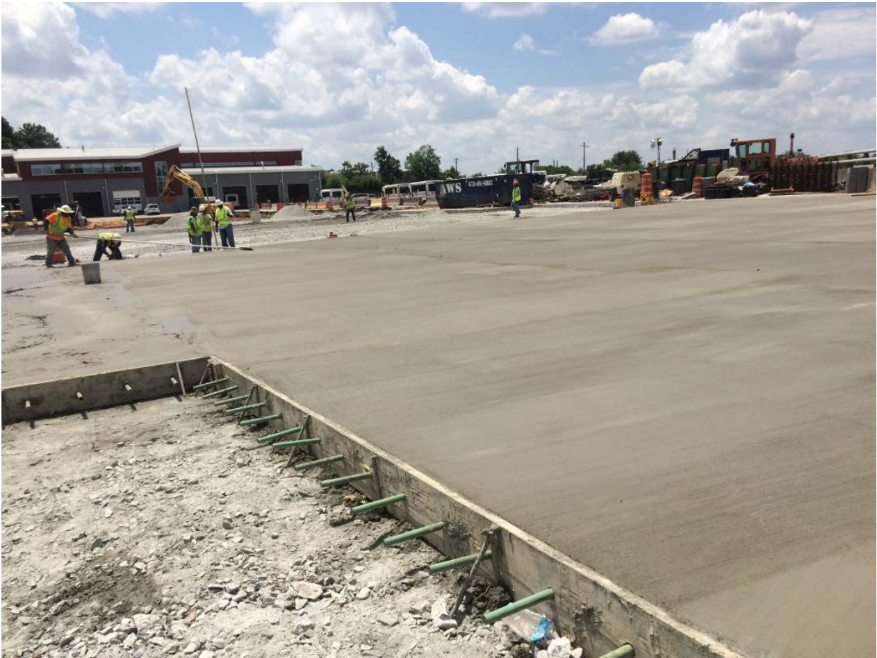
Figure 2. EdenCrete™ enriched slab being installed
