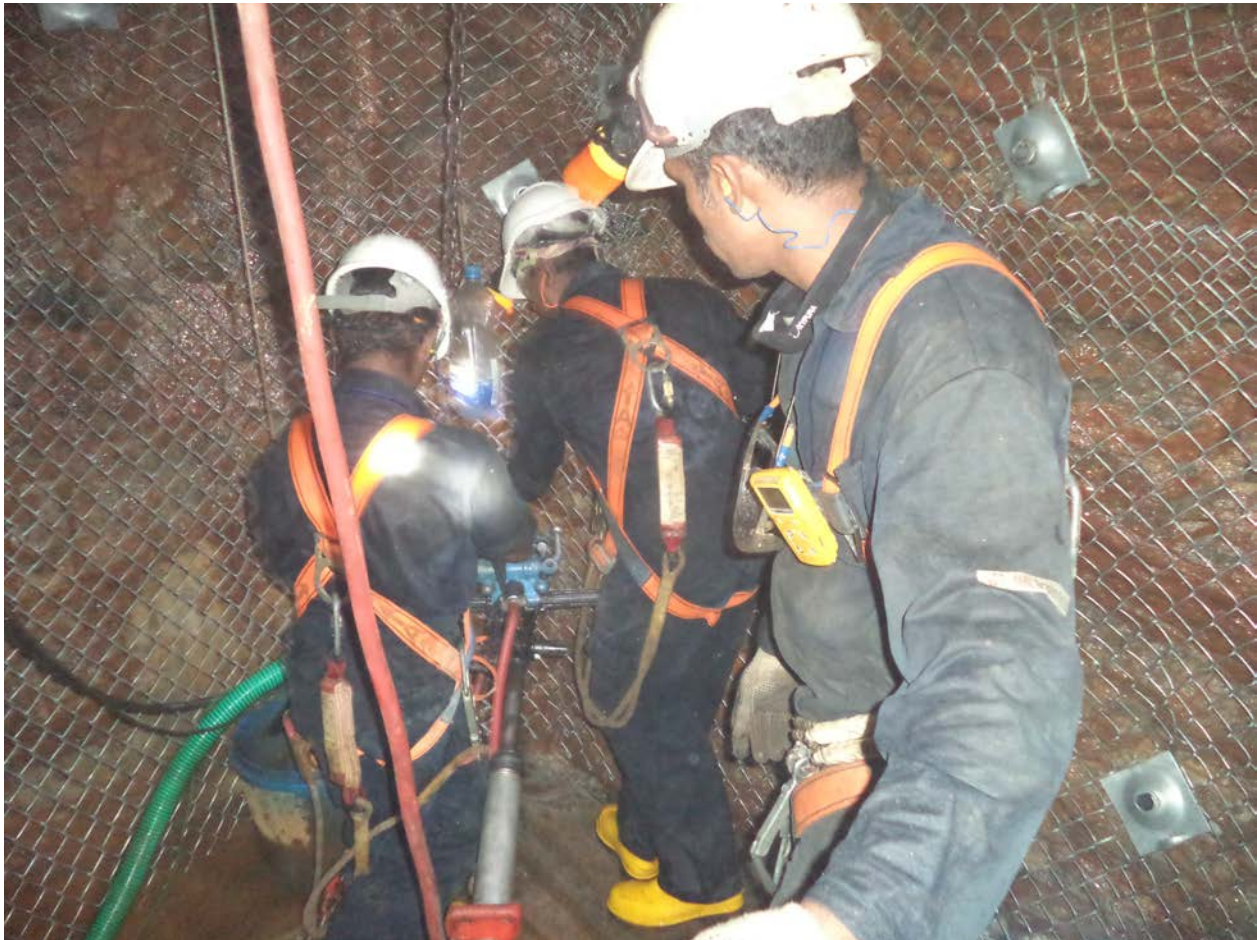
Figure 3: Miners installing mesh and bolt support in the Pandeniya shaft
