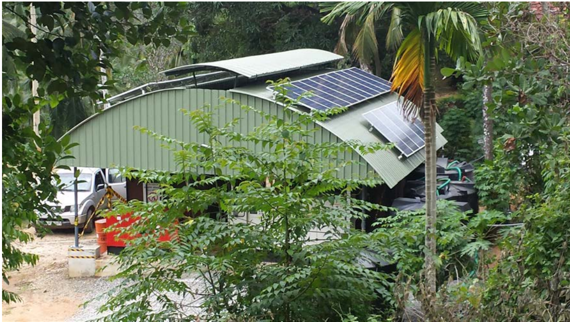
Figure 4: Pandeniya workshop and office facilities with solar power and battery storage
