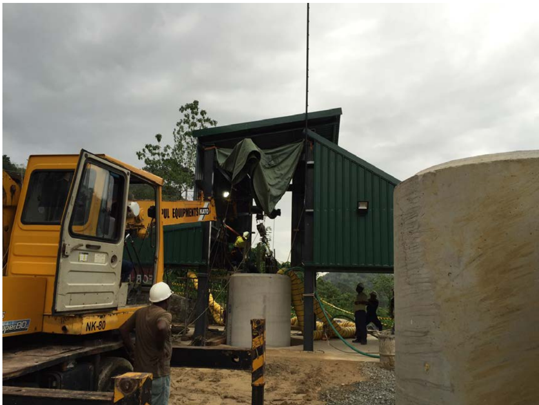
Figure 5: Installation of liner seven at Aluketiya Shaft H
