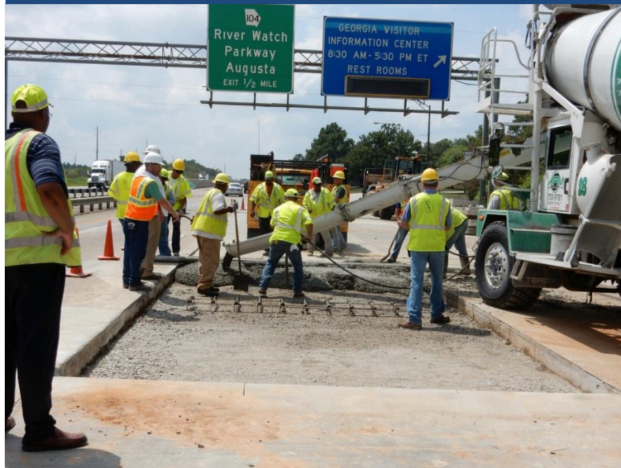
Picture from August 2015 GDOT I-20 Field Test
