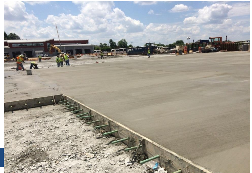
EdenCrete™ Trial Slab
