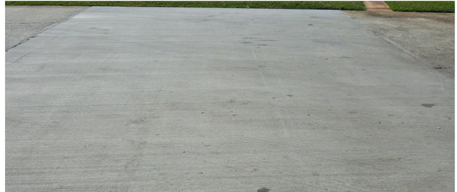
EdenCrete™ Trial Slab after 6 months No cracks or evidence of wear
