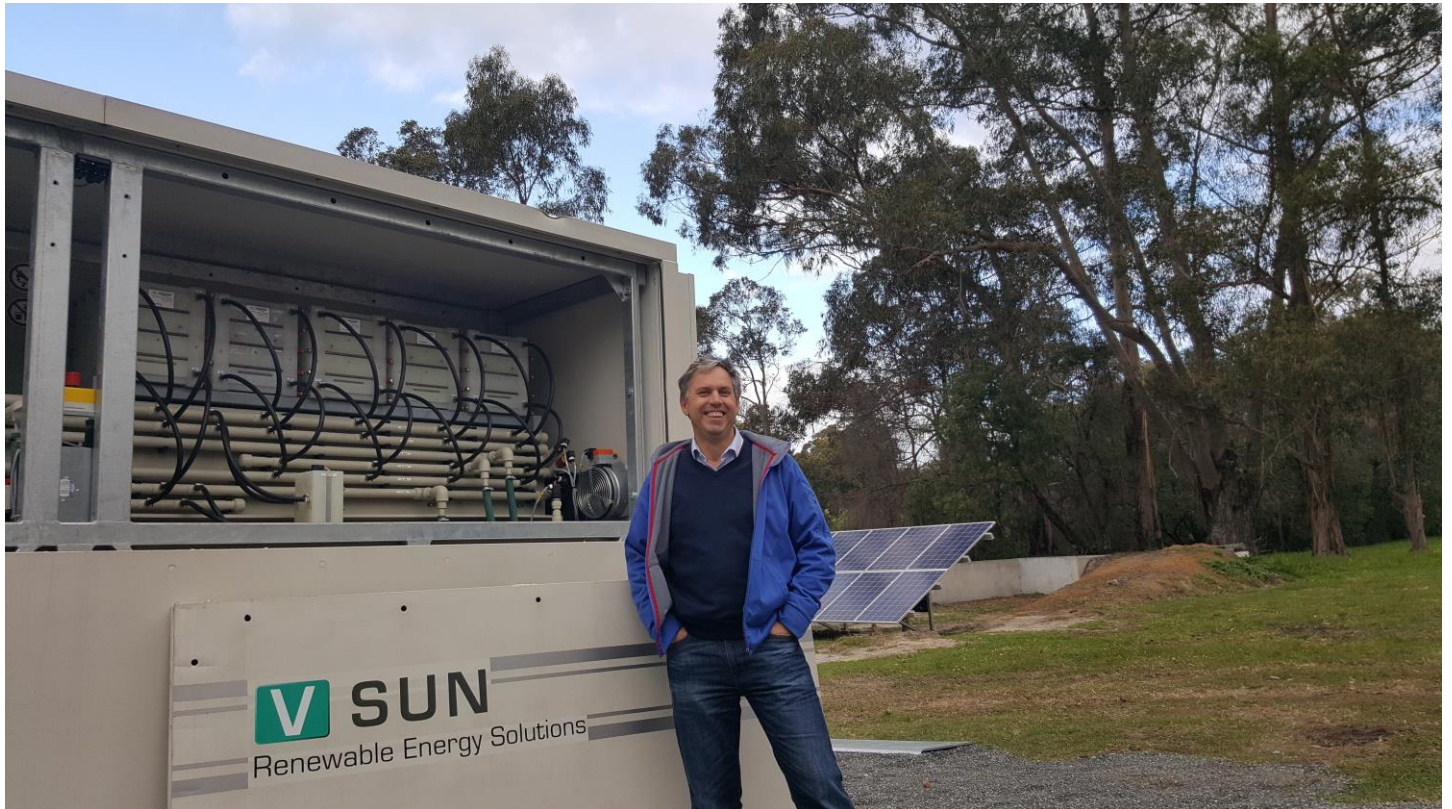
Managing Director, Vincent Algar, next to the CellCube vanadium redox flow battery.
