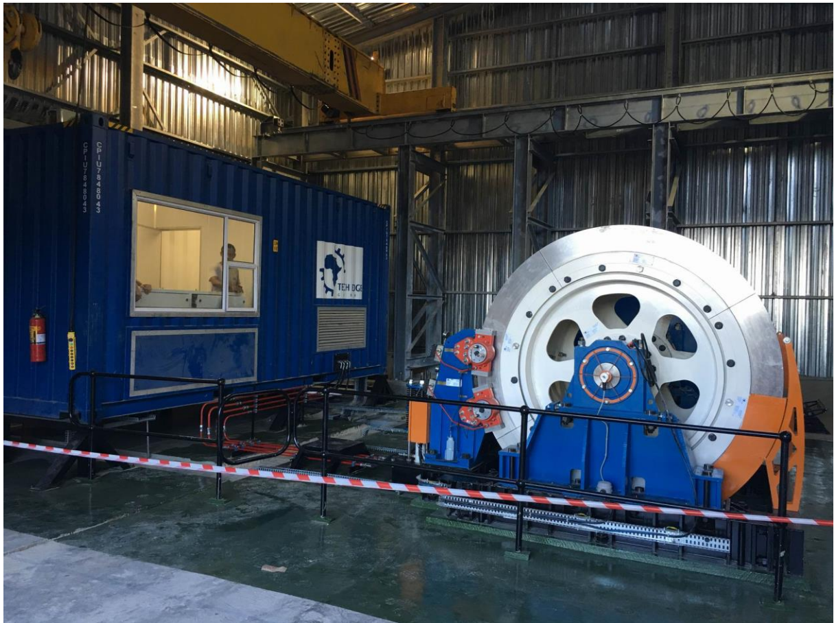
Photo 1. E15 Service Shaft Main Winder
