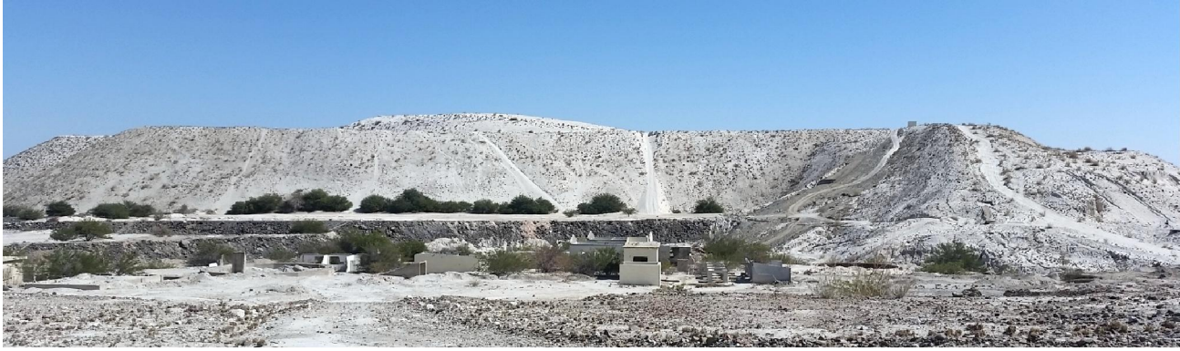
Photo 1 | Course sands stockpiles up to 60m high
