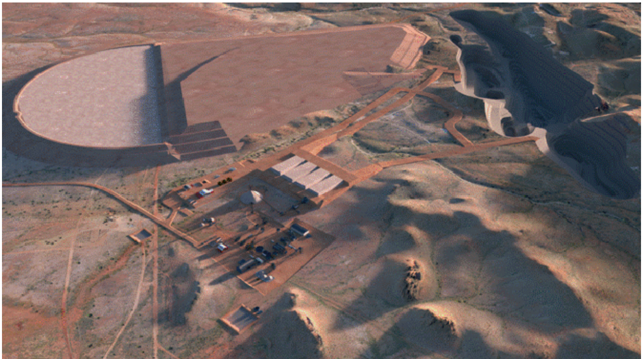
Figure 9 – Altura Pilgangoora Lithium Project – Pit - Waste Rock Dump and TSF 3D Model
