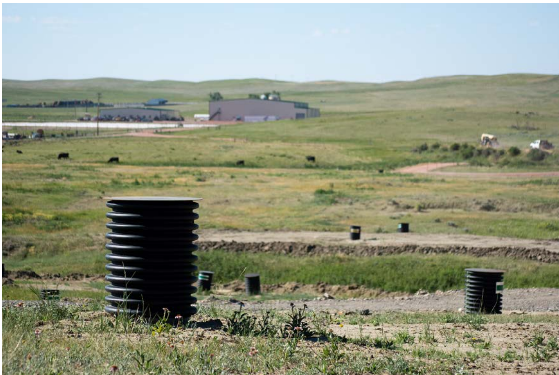
Figure 4: Well fields (CPP and Admin Building in background), Lance Projects – June 2016
