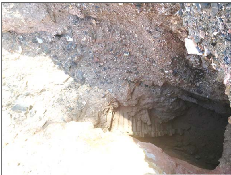
Photo 4: Merry Hamptons with wooden pillar to support back-filled stope
