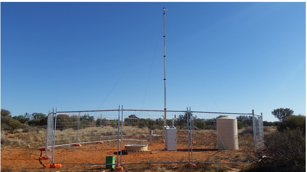
Figure 9 – AWS Installed at Lake Wells
