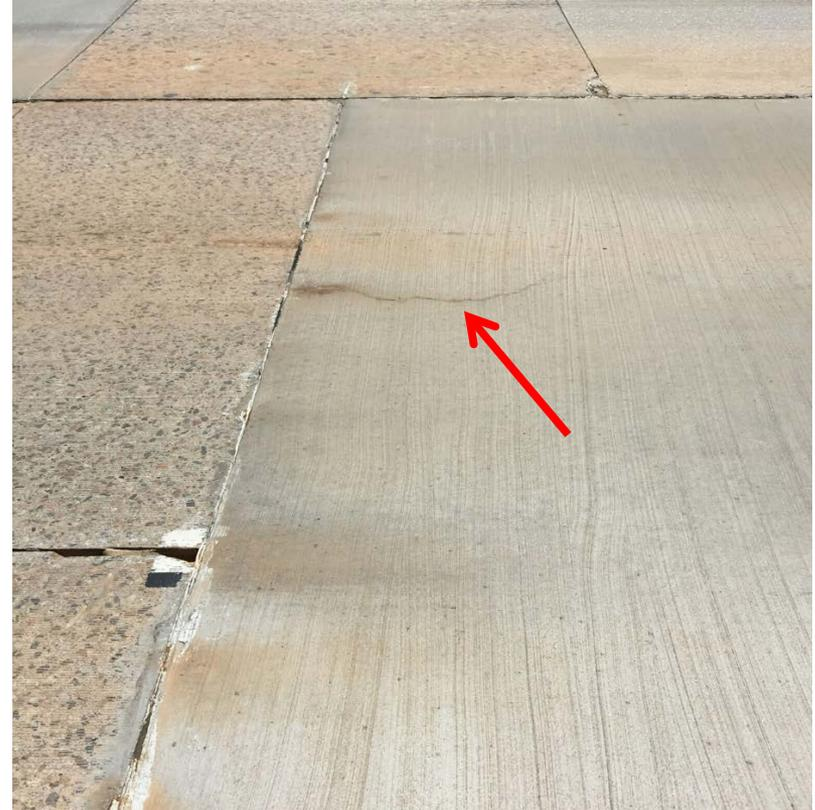
**Control - Visible Crack Developing**
