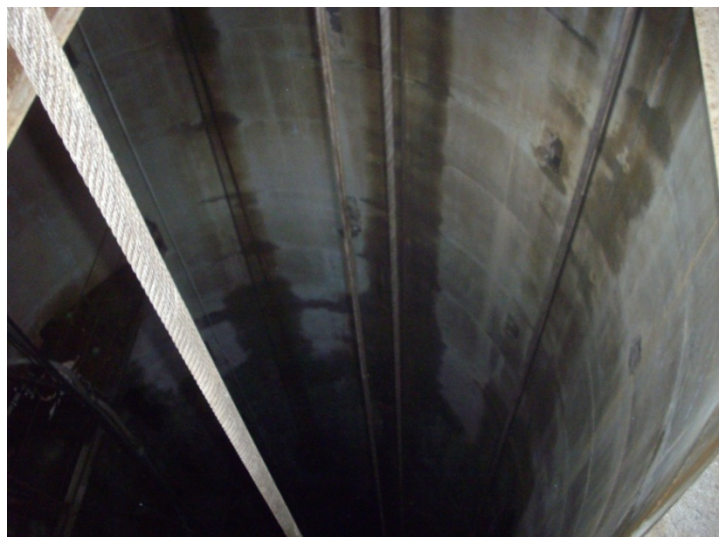
Shaft 5: Photo taken at Shaft 5 collar looking down at the lined 7m diameter shaft
