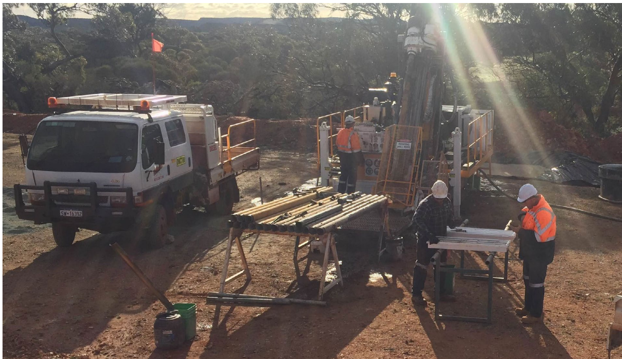
Figure 7: Diamond Drilling at Mulgine Hill – August 2016
