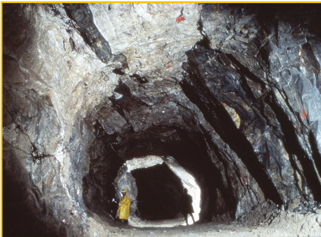
Figure 7: Photo of Underground Workings at Wolfsberg.
