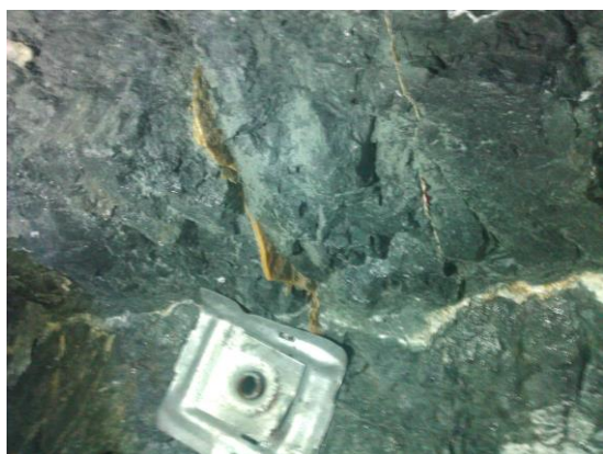
Image 3 – Chemical resin post grouting
