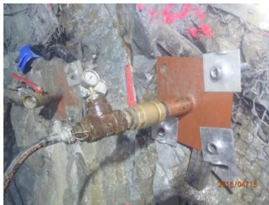
Image 2 – Cement pre grouting
