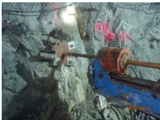
Image 1- Cement pre grouting
