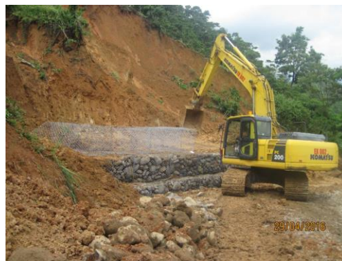
Image 7: Erosion control in areas affected by landslides
