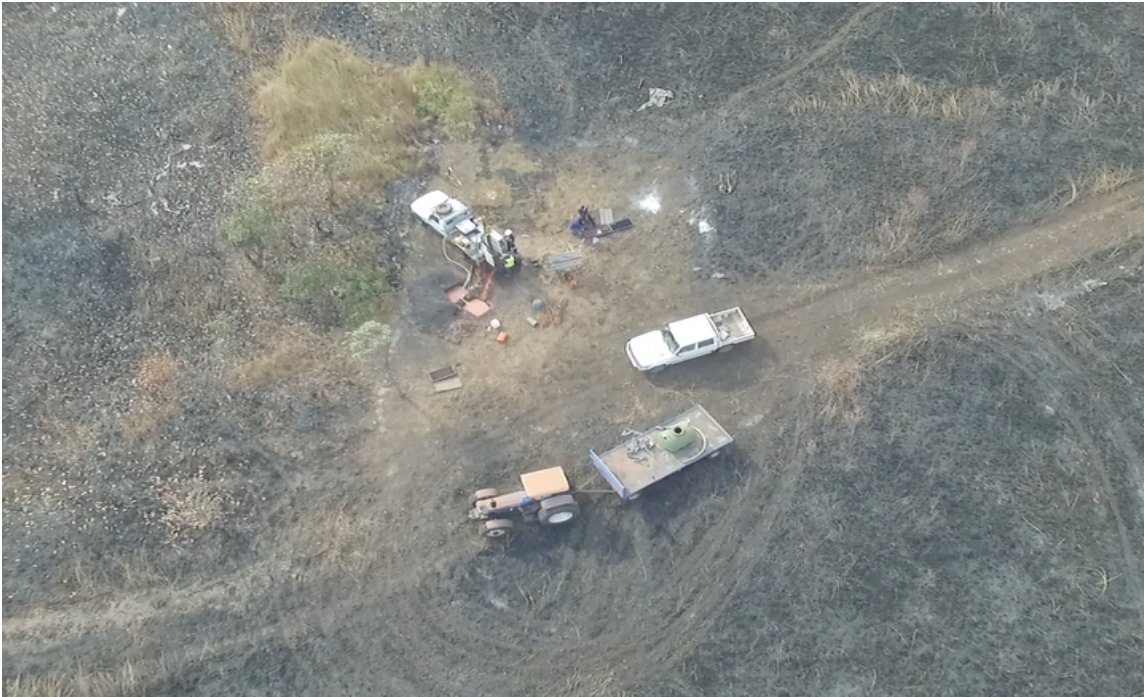
Core drilling of L259 with the mobile Sedidrig rig
