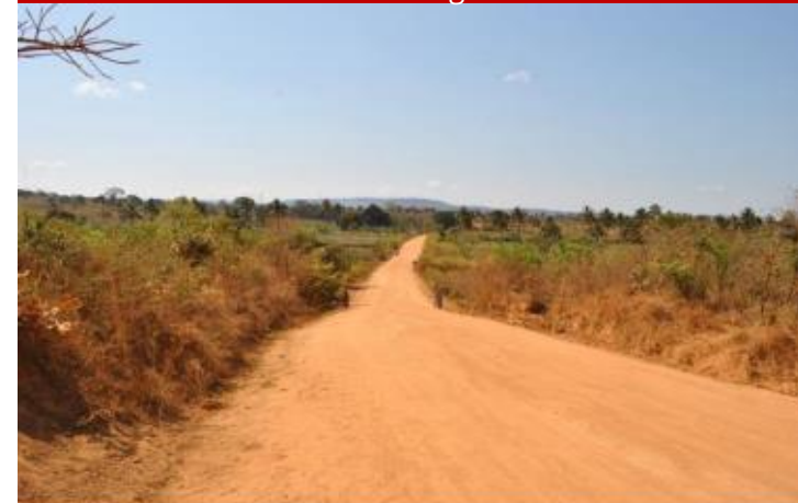
Typical section of flat lying road between Nanganga and Ruangwa
