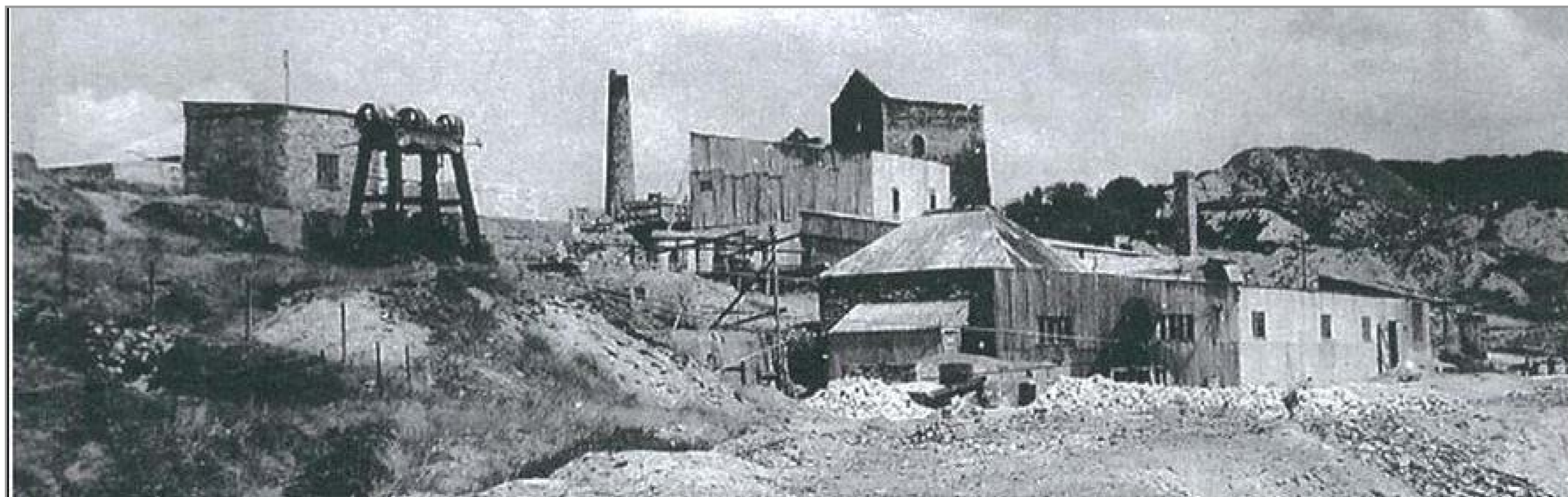
Redmoor Processing Plant circa 1920's
