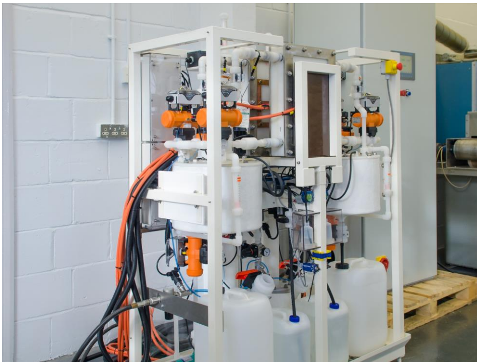
Example of a pilot electrolyte preparation plant
