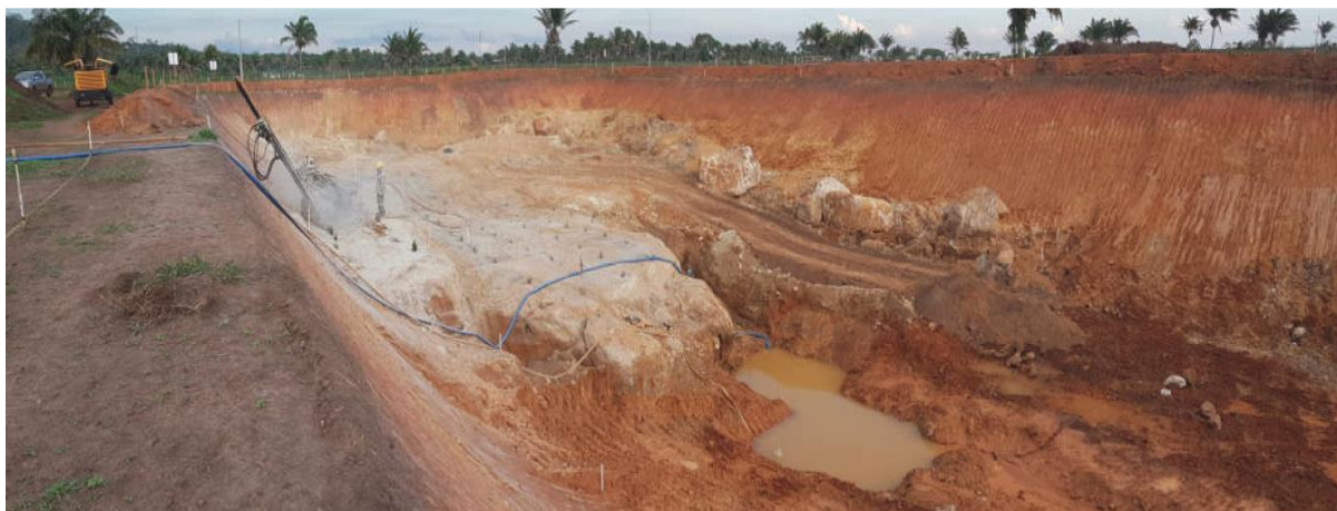
Drilling in progress within the Pedra Branca box-cut
