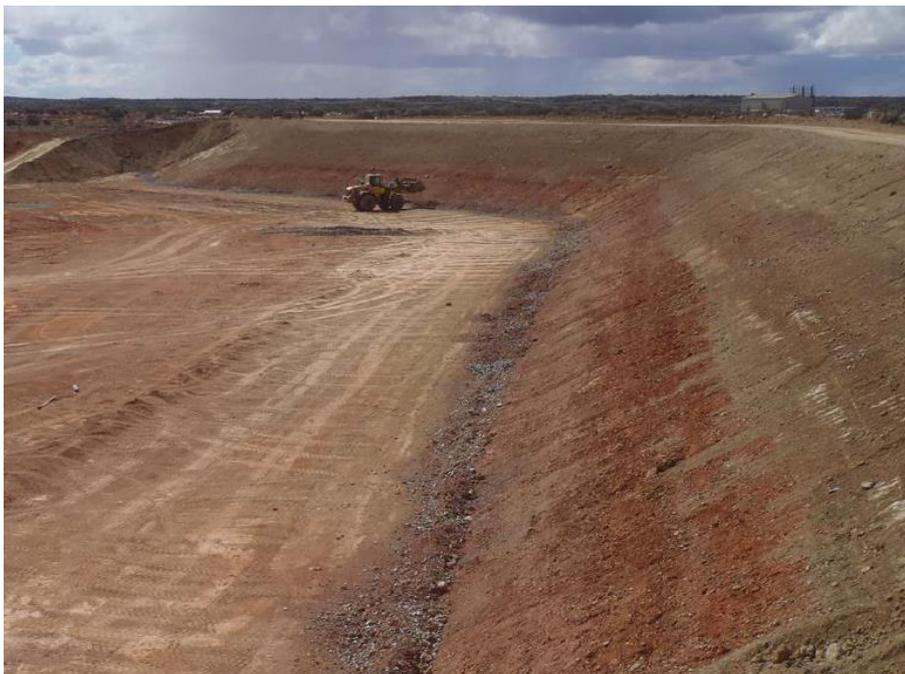
**Photo 7: New TSF Dam ready for discharge**
