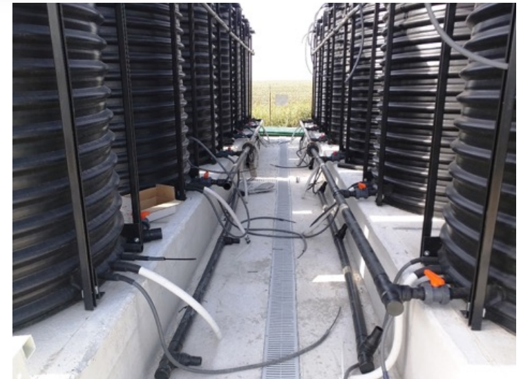
Final construction steps in progress
