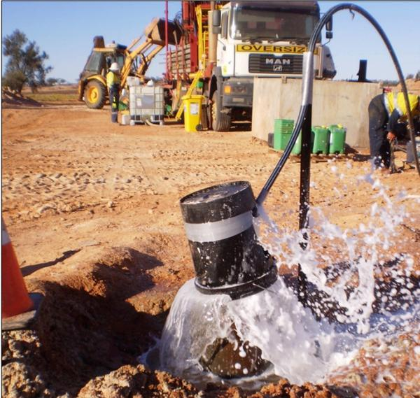
Figure 6: Sourcing well-development water from test-production bore #1 Site A
