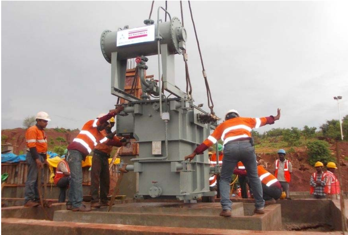
Transformer Erection
