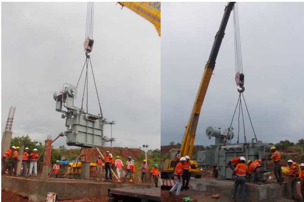
Transformer Unloading and Erection
