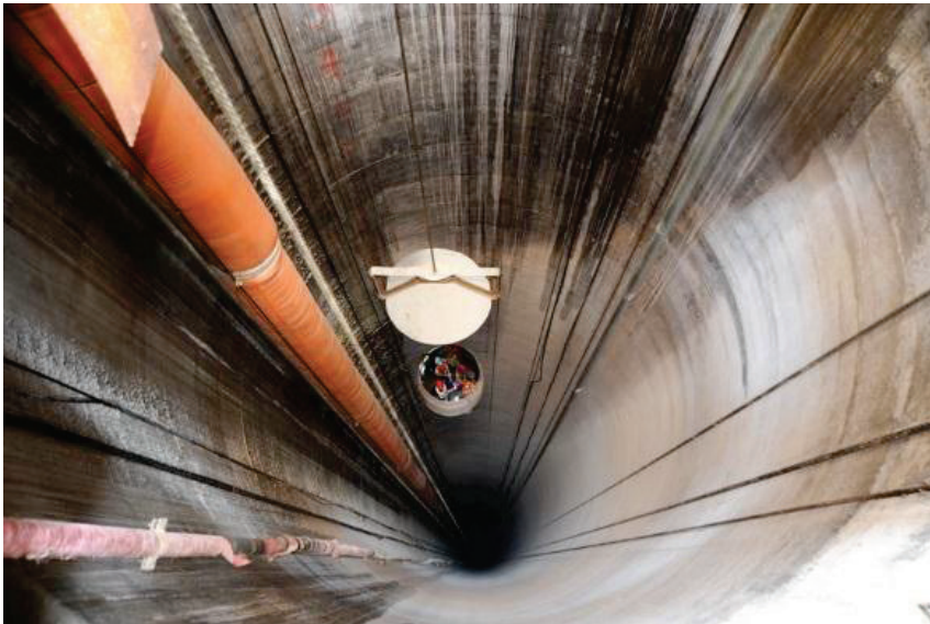
Figure 2 – Nalinhe 8 Mtpa Coal Mine Shaft – CC5C project utilizing ground freezing
