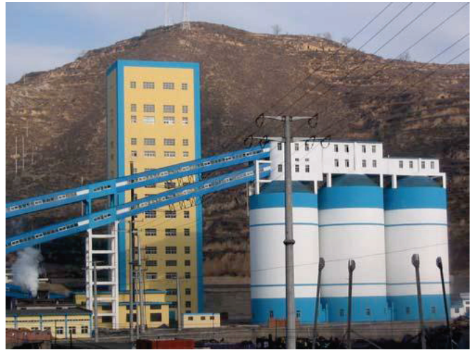
Figure 7 – Asia's tallest shaft tower constructed by CC5C
