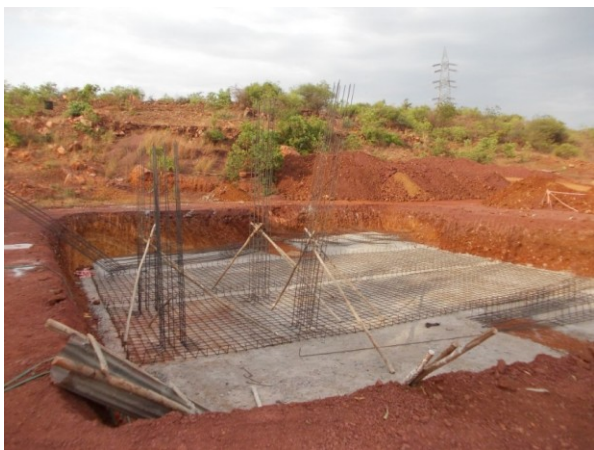
Foundation works concreting commencement
