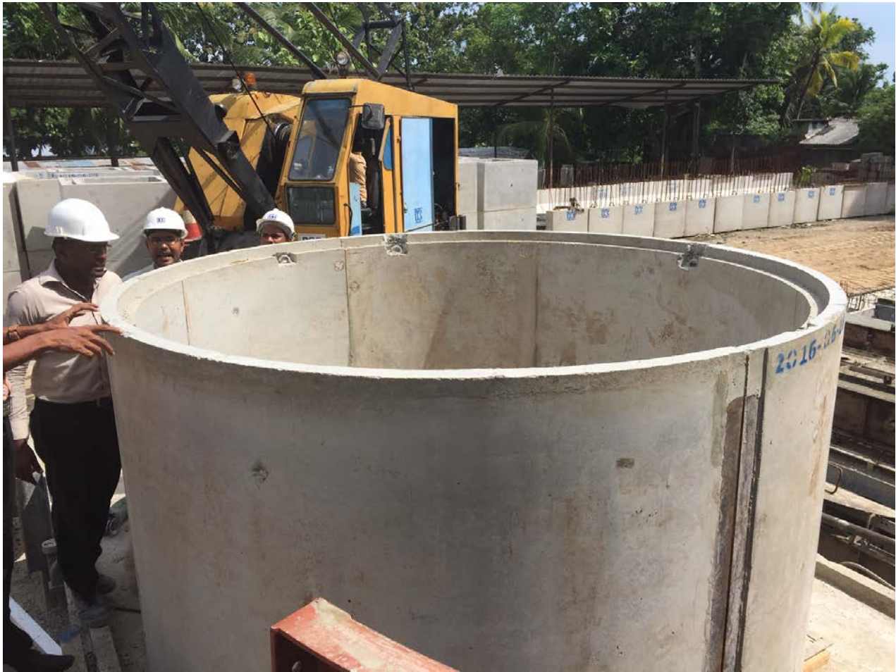
Figure 6: First trial set of 2.5m diameter shaft liners for Shaft J from FGR designed mould
