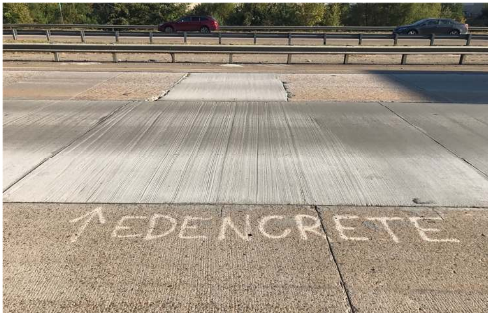
Figure 2. EdenCrete™ trial slab on I-20 Field trial showing no cracking or visible wear after 14 months.
