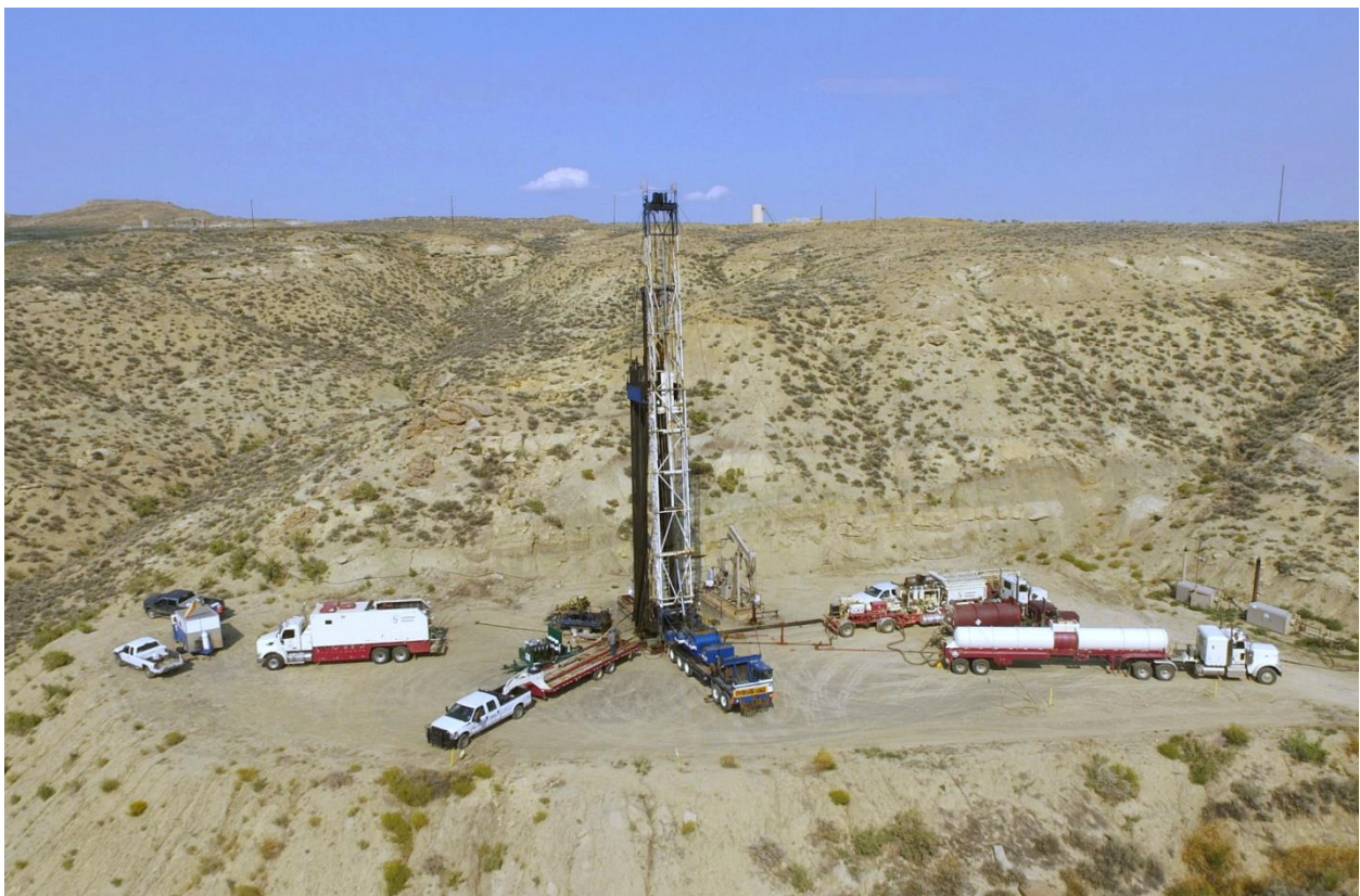
Well recompletion rig and ancillary equipment, Silvertip Field
