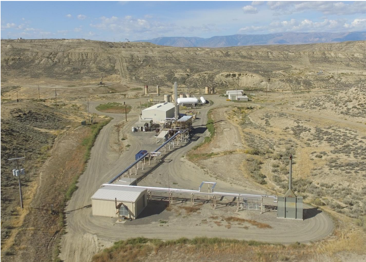
Incremental's wholly owned Gas Processing Plant, Silvertip
