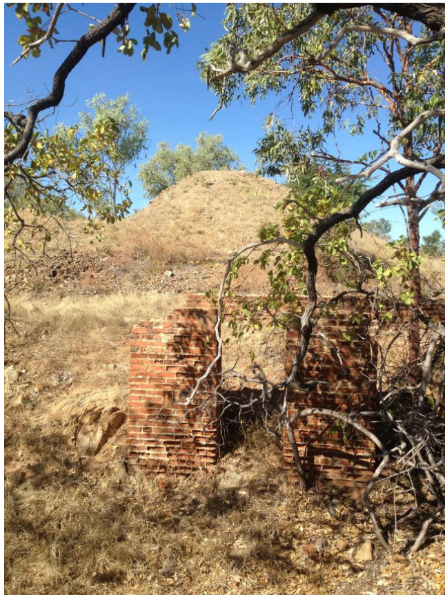
Photo 12: Nil Desperandum main shaft showing probable winder foundations
