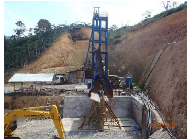
Completed Headframe for 5 Level shaft
