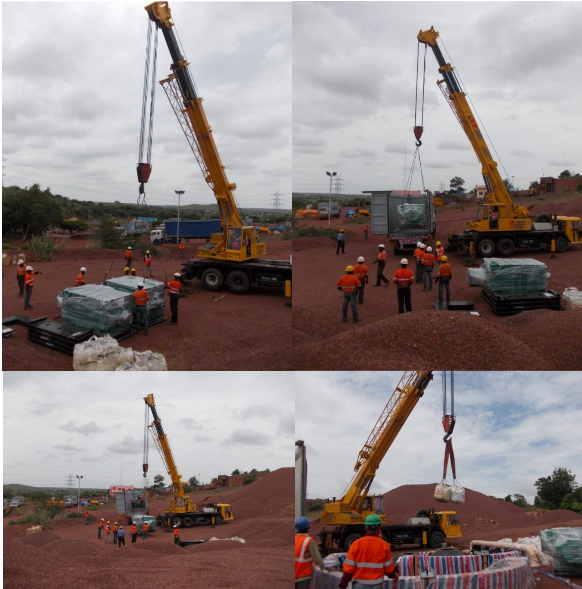
Chinese equipment unloading adjacent to wet plant feed stockpiles
