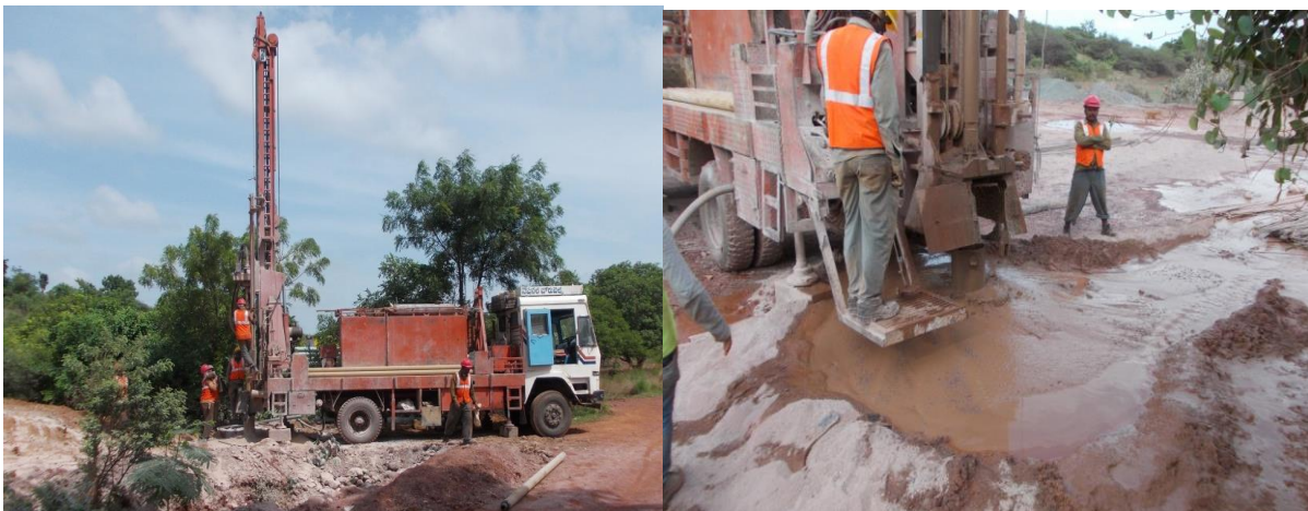
Bore well drilling
