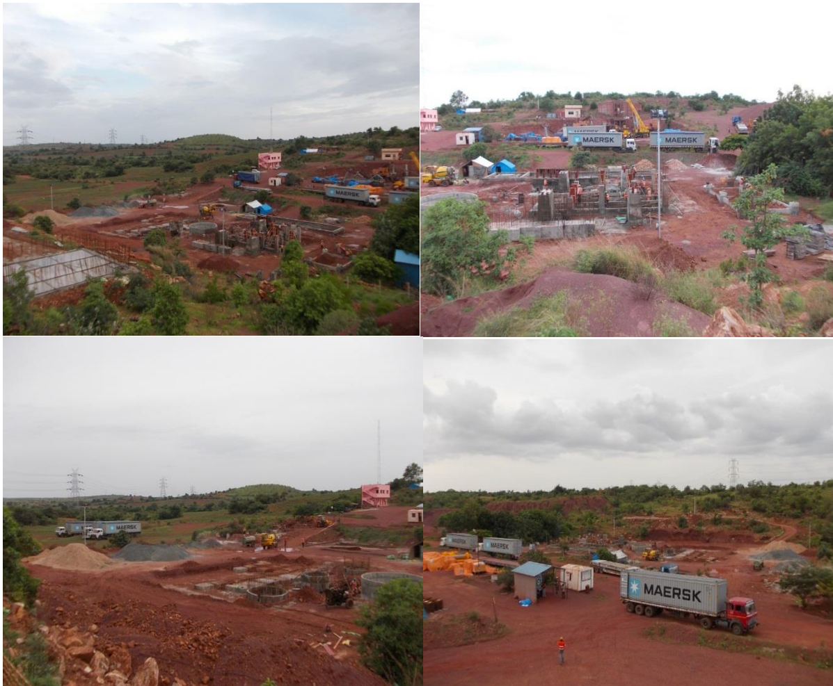
Third Chinese equipment shipment arriving on site
