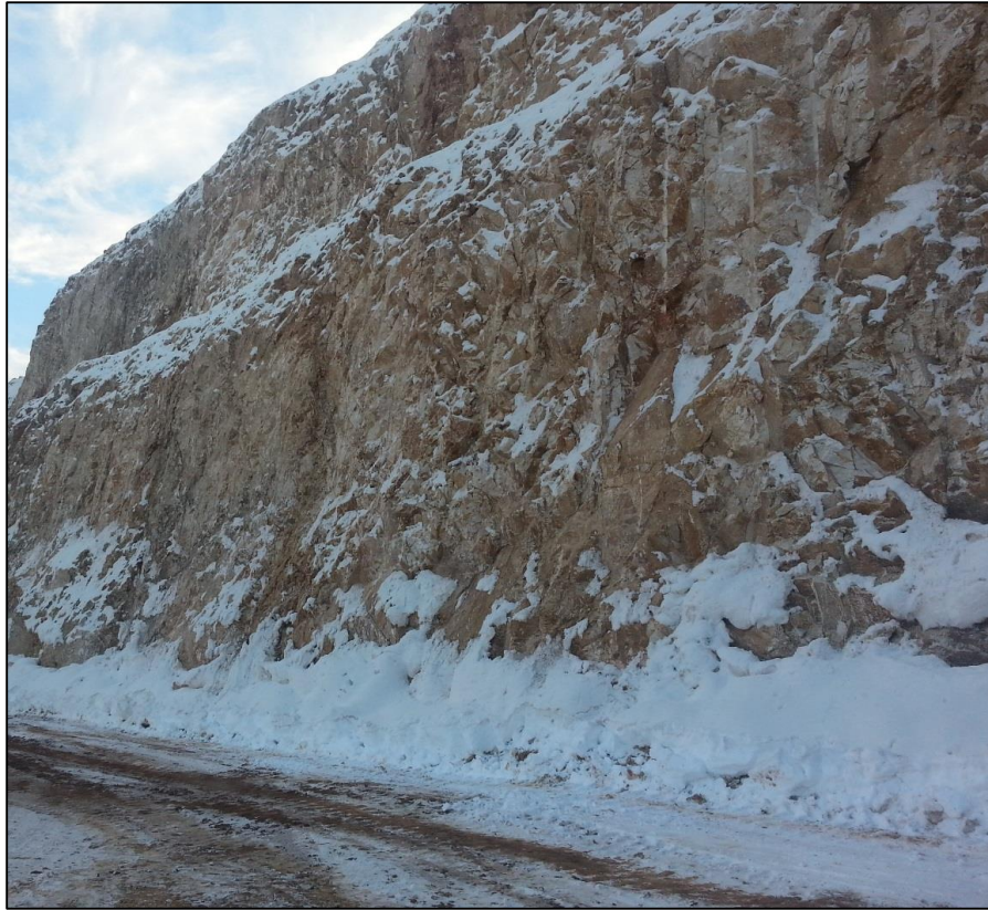
Figure 16-4 Typical 15 m pre-split at Çöpler Mine
