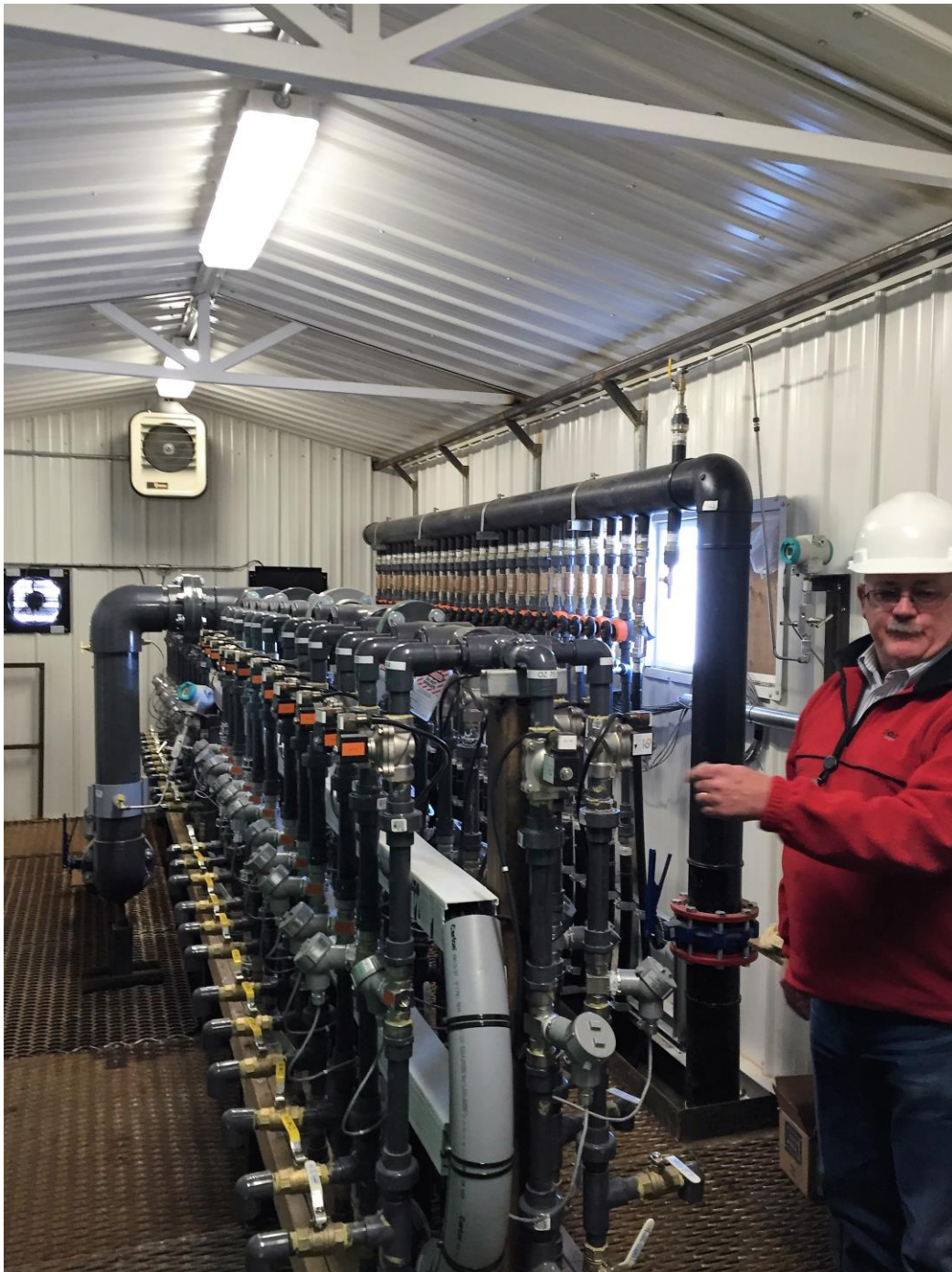
Figure 3: Header House, Lance Projects – April 2016
