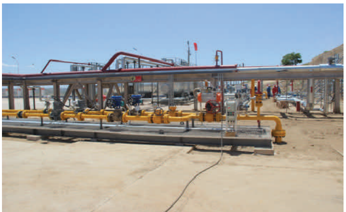
New Metering Skid at Linxing CGS for sales to Huasheng
