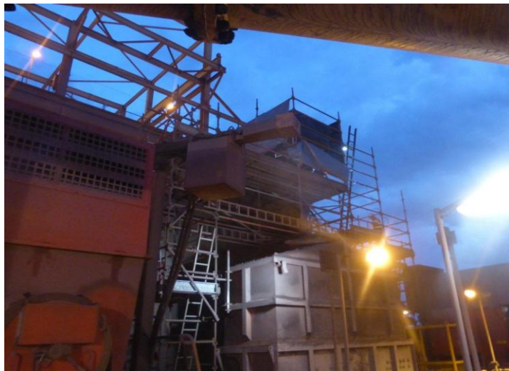
Scaffolding set up to enable access for repairs of the SAG mill girth gear
