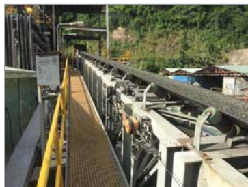
Mill feed conveyor
