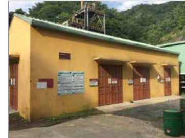
Mill and process plant LV substations
