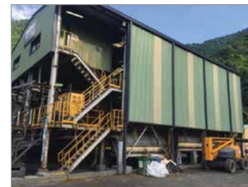
Flotation building with control room
