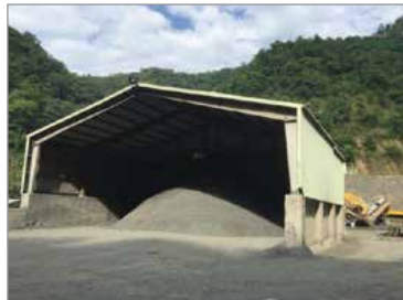
Fine ore shed
