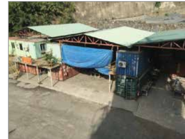
Office and workshop complex
