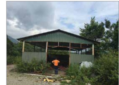
Disused warehouse near upper portal
