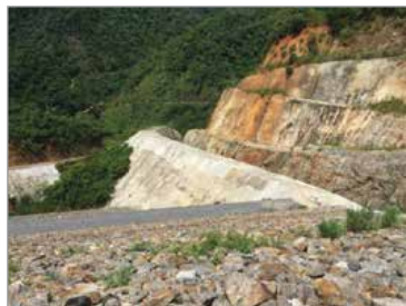
The TSF spillway
